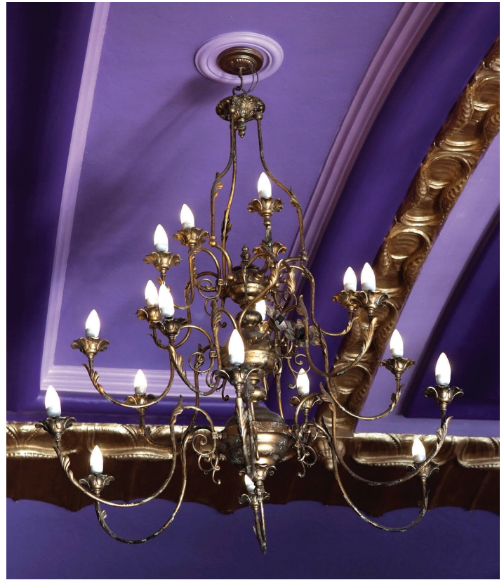
Hamburger Mary’s uses 48 cold-cathode, dimmable, fluorescent lamps in its three upstairs chandeliers.
